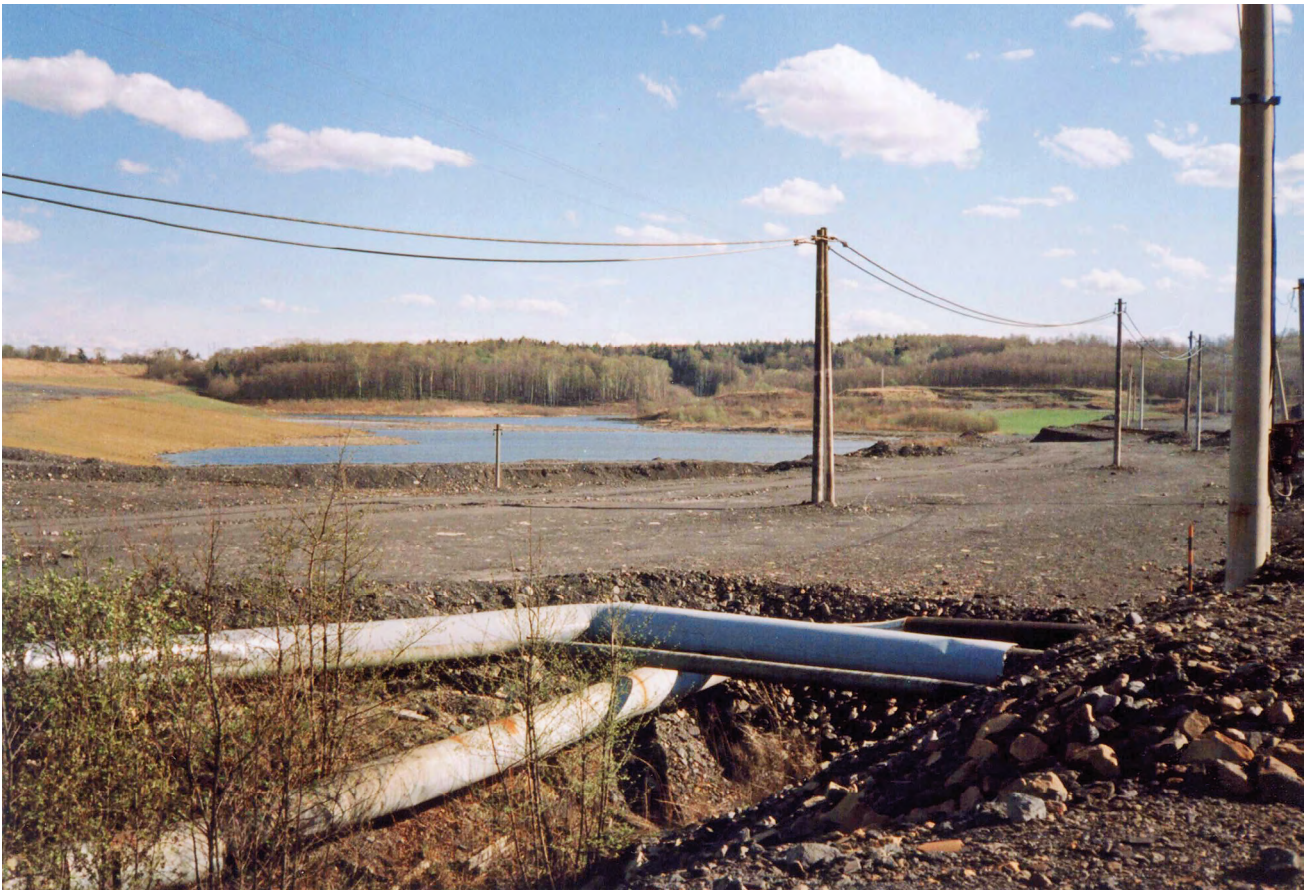
Fig. 24 Ground subsidence (Lazy mining area). Photo: M. Mulková, 1998
