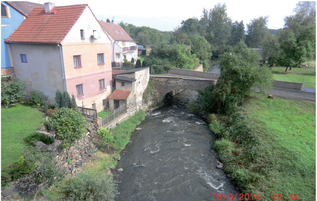
Fig. 9 The urban village of Rtyně nad Bilinou. Reach BIL019, inappropriately placed buildings directly on the edge of the watercourse. In combination with reduced throughput caused by narrowing the channel profile bridge, high water flows could threaten buildings along the river channel.
