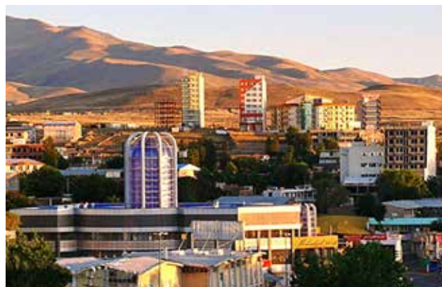
Fig. 11 Another view of construction in the city of Sarein after the 1997 earthquake.
