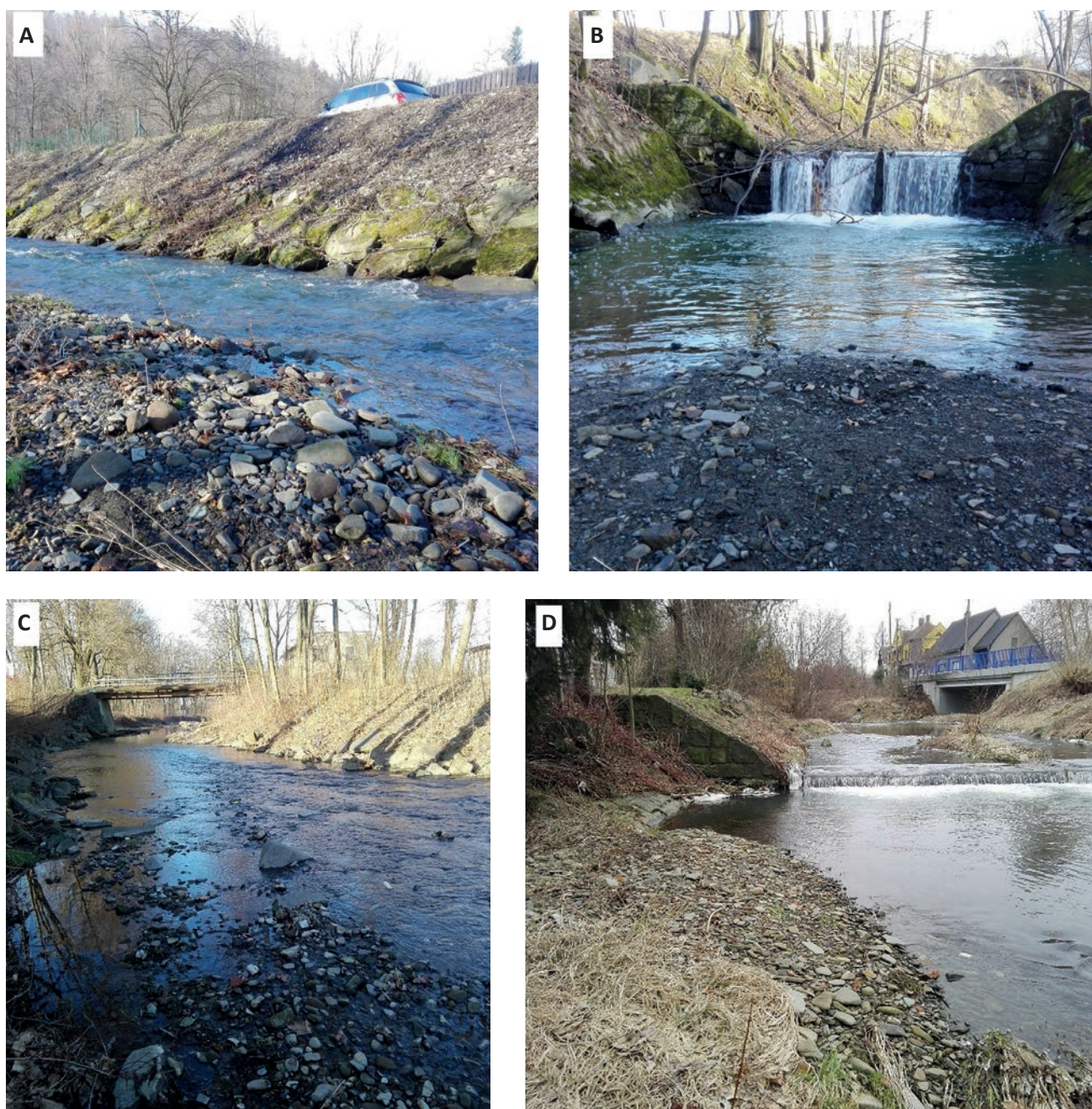
Fig. 2 Examples of previous river regulations; (A) large rocks (riprap) along the levee on right bank (the Lubina, channel width = 8 m, left-side bar, curved section); (B) check dam (the Lubina, channel width = 9 m, mid-channel bar, curved section); (C) bridge construction (the Ondřejnice, channel width = 11.5 m, left-side bar, straight section); (D) stone rockfill and grade control structure (the Ondřejnice, channel width = 11.5 m, right-side bar, straight section). Source: Author.
