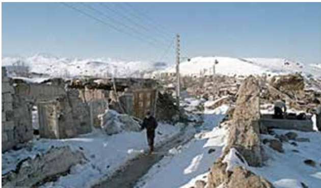
Fig. 8 An overview of the earthquake that occurred in 1997 in Sarein.
