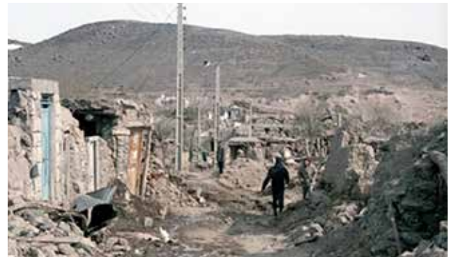
Fig. 9 An overview of the earthquake that occurred in 1997 in Sarein.
