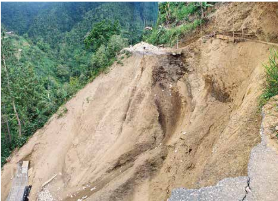
Fig. 3 Landslide on the B1 road at Section in Portland Parish, Jamaica. This event severed much of the local coffee production industry from the ports used to ship the product to market. (The picture is a photo-collage and some distortion is inevitable.)
