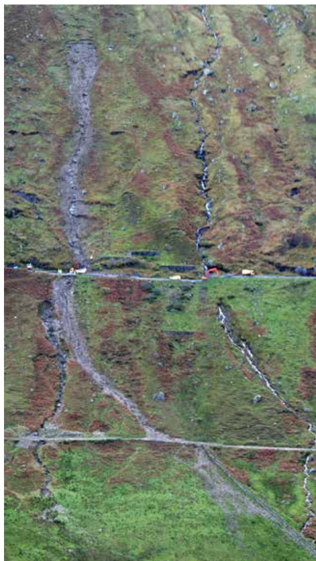
Fig. 2 View of the debris flows above and below the A83 on the approach to the Rest and be Thankful (location approximately that of 1b in Figure 1). The head scar is at approximately 370 m Above Ordnance Datum (AOD), the A83 at 240 m AOD and the Old Military Road (OMR) at 180 m AOD.
